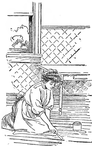
"The Cracks May be Filled."
