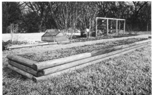
B. Reinforcing Rods Hold Timbers Together.
