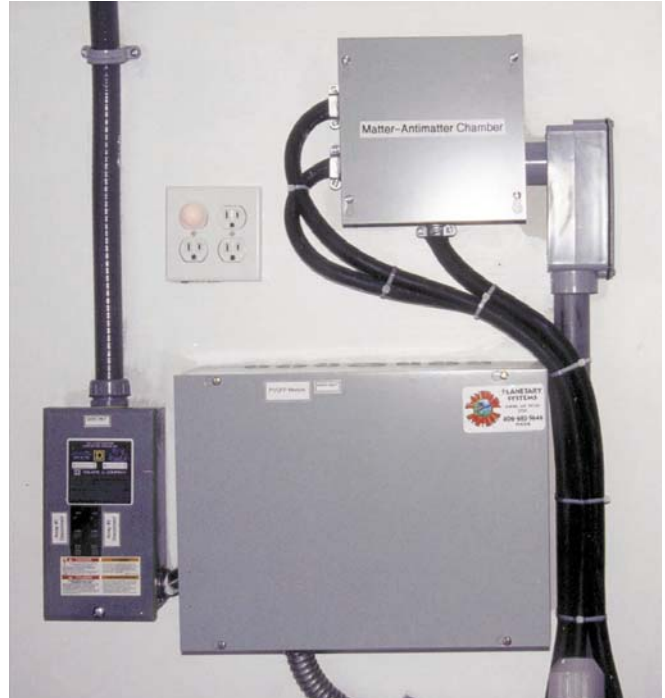
Solar array 40 amp breakers and Trace PVGFI-2 ground fault interrupter.
