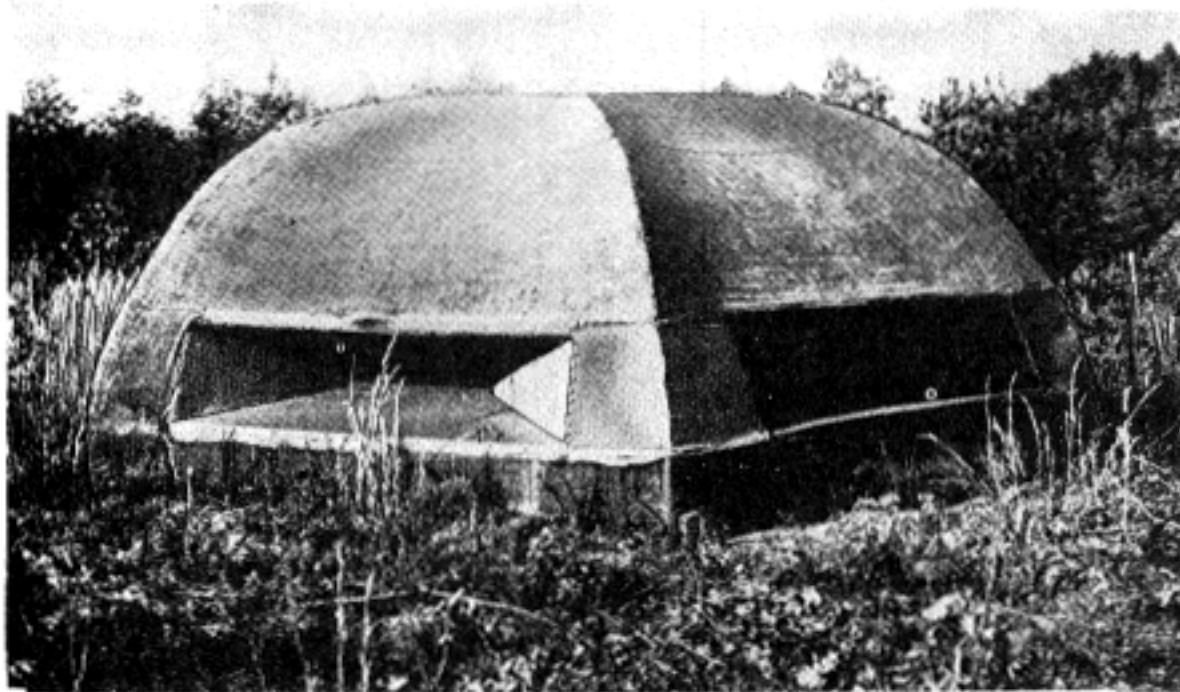
Figure 75. Here is a decoy pillbox constructed of wood, covered with burlap or osnaburg, and sprayed with paint to resemble concrete. Sand and dirt may be sprinkled on the wet paint to give it a concrete-like texture.
