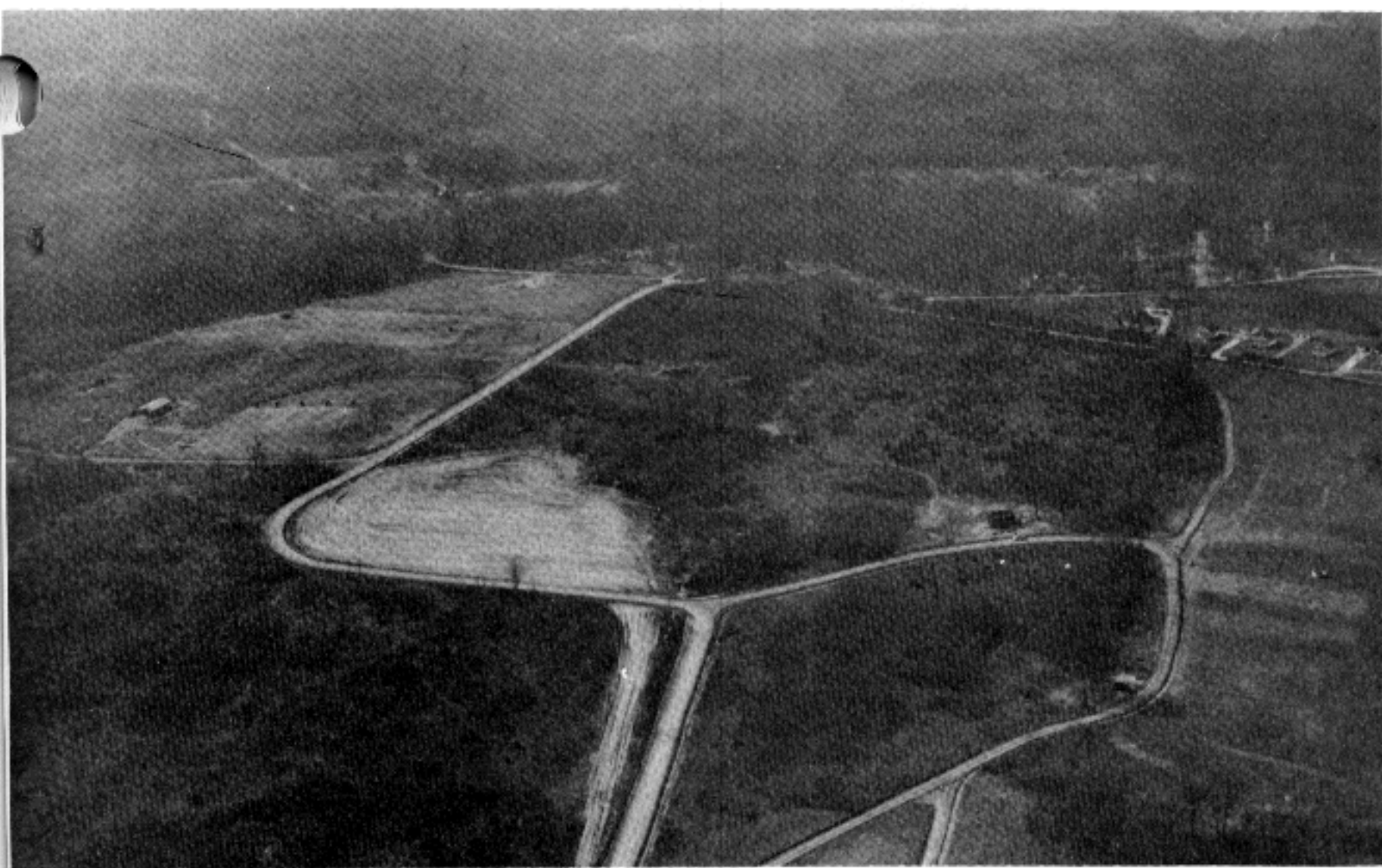
Figure 54. Careless and widespread earth scarring is caused by failure to establish a traffic plan, indiscriminate use of earthmoving equipment, and too much concern with leveling and clearing to facilitate construction. An enforced traffic plan, set up during the planning stage would eliminate much of the revealing scars in this picture.
