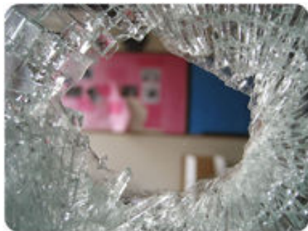
FIGURE 1: When glass breaks, its physical properties change. Instead of one solid sheet of glass, it now has holes and cracks.
