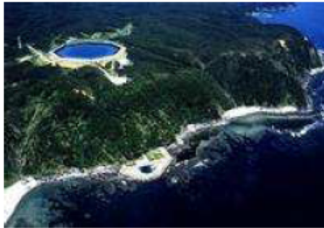
Figure 26.11: Okinawa pumped-storage power plant, whose lower reservoir is the ocean. Energy stored: 0.2 GWh. Photo by courtesy of J-Power. www.ieahydro.org .
