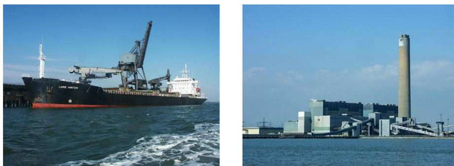
Figure 23.1: Coal being delivered to Kingsnorth power station (capacity 1940 MW) in 2005. Photos by Ian Boyle www.simplonpc.co.uk .
