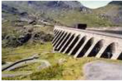
Figure 26.6: Llyn Stwlan, the upper reservoir of the Ffestiniog pumped storage scheme in north Wales. Energy stored: 1.3 GWh. Photo by Adrian Pingstone.
