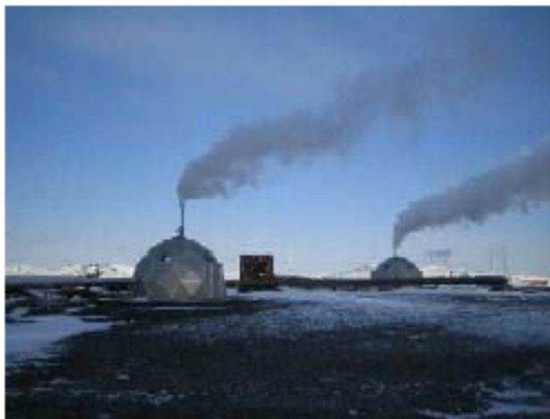
Figure 25.11: More geothermal power in Iceland. Photo by Rosie Ward.
