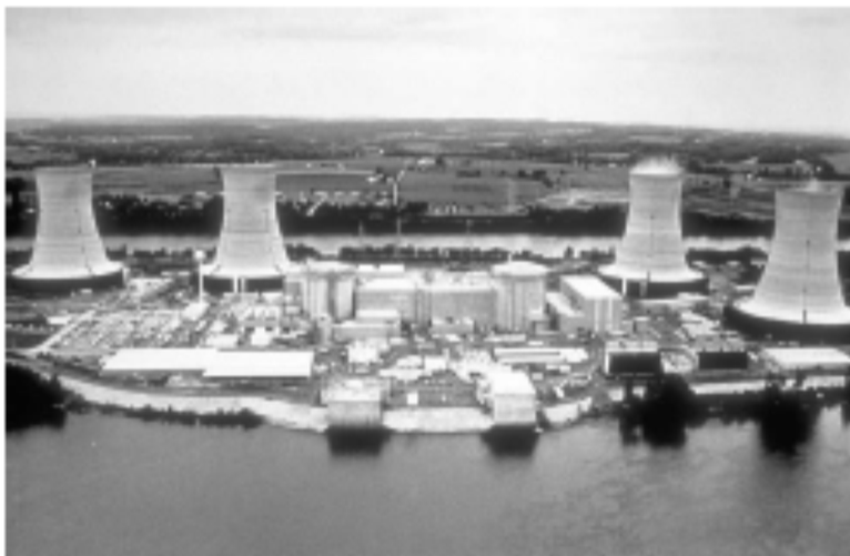
Figure 24.4: Three Mile Island nuclear power plant.
