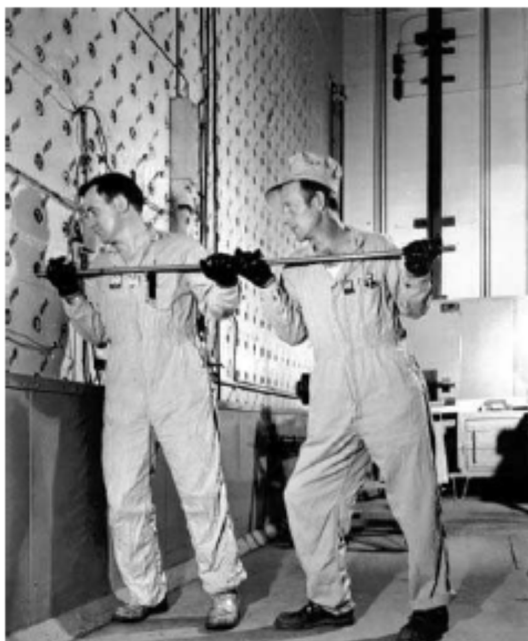
Figure 24.3: Workers push uranium slugs into the X-10 Graphite Reactor.
