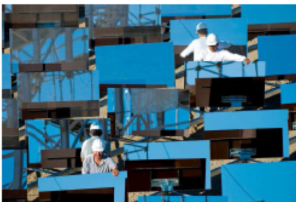
Figure 25.12: Two engineers assembling an eSolar concentrating power station using heliostats (mirrors that rotate and tip to follow the sun). esolar.com make medium-scale power stations: a 33 MW (peak) power unit on a 64 hectare site. That's 51 \text{ W}/\text{m}^2 peak, so I'd guess that in a typical desert location they would deliver about one quarter of that: 13 \text{ W}/\text{m}^2 .
