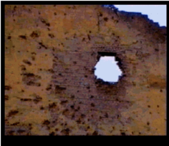
Figure 7-19. Examples of penetration and damage to buildings.
