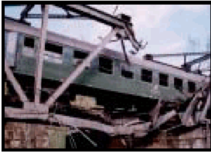
Figure 7-24. Example of a damaged rail transportation system.
