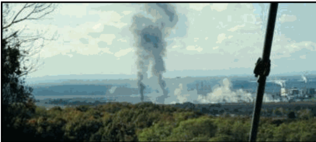
Figure F-7. Petrochemia chemical plant under attack by Serbian forces.
