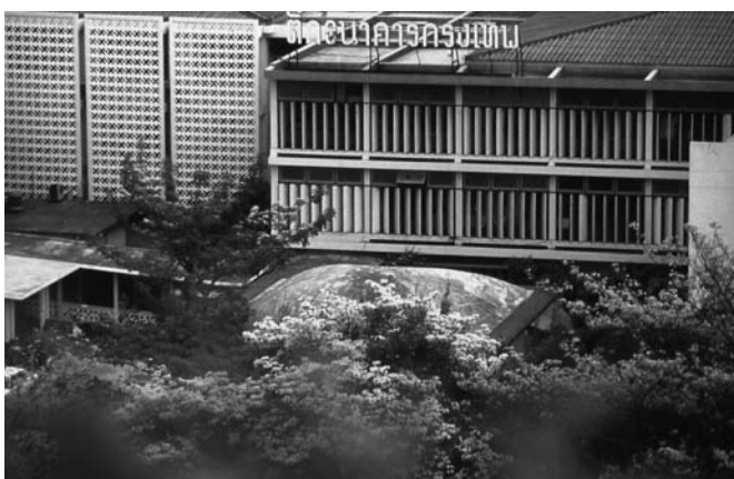
Figure 19.3 The Bangkok Bank Building, ideally designed for neurology, neurosurgery, and psychiatry services on each floor in its three-storied structure was opened in 1960. Early neurosurgery, of the 1960s to modern epilepsy surgery of the 21st century took place here in its long evolutionary history. Now the location of the Chulalongkorn Comprehensive Epilepsy Program.
