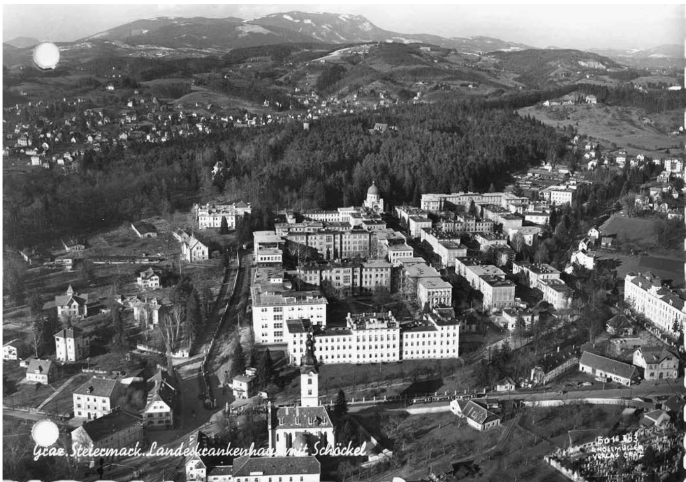
Figure 8b.2 (a) Historical view of the Landeskrankenhaus Graz.
